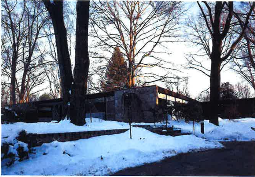
Front Entrance from driveway
