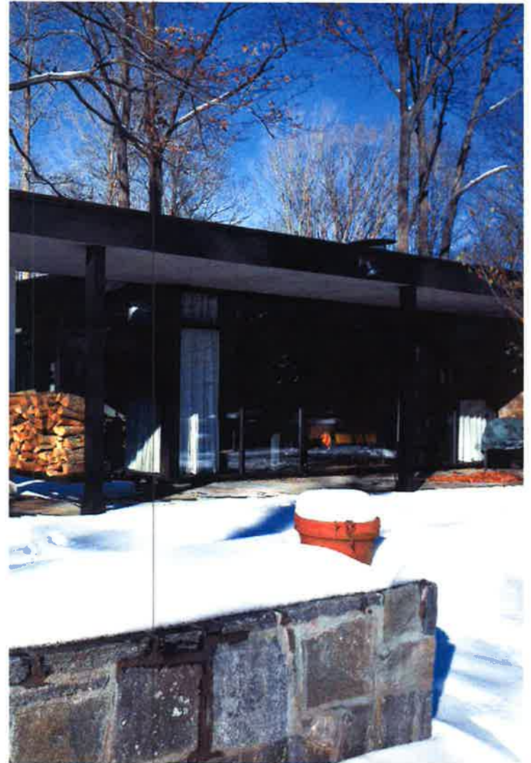
Main Patio outside of Living Room
